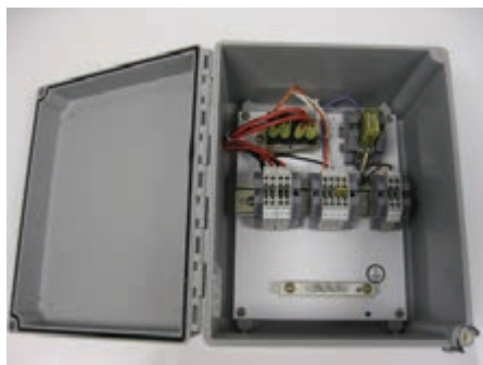
Dump Pump Contractor Panel
